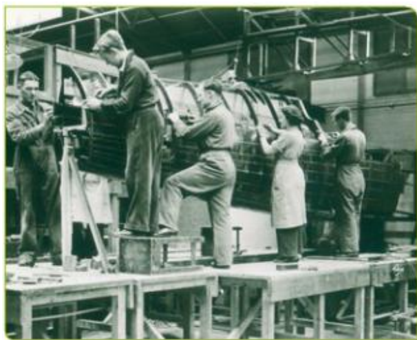
The first composite aircraft fuselage, built for a Spitfire in 1940 by Hexcel's UK site
